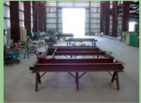
The Base Fabrication Area covers 15,000 square feet and is fully equipped for speed and accuracy
